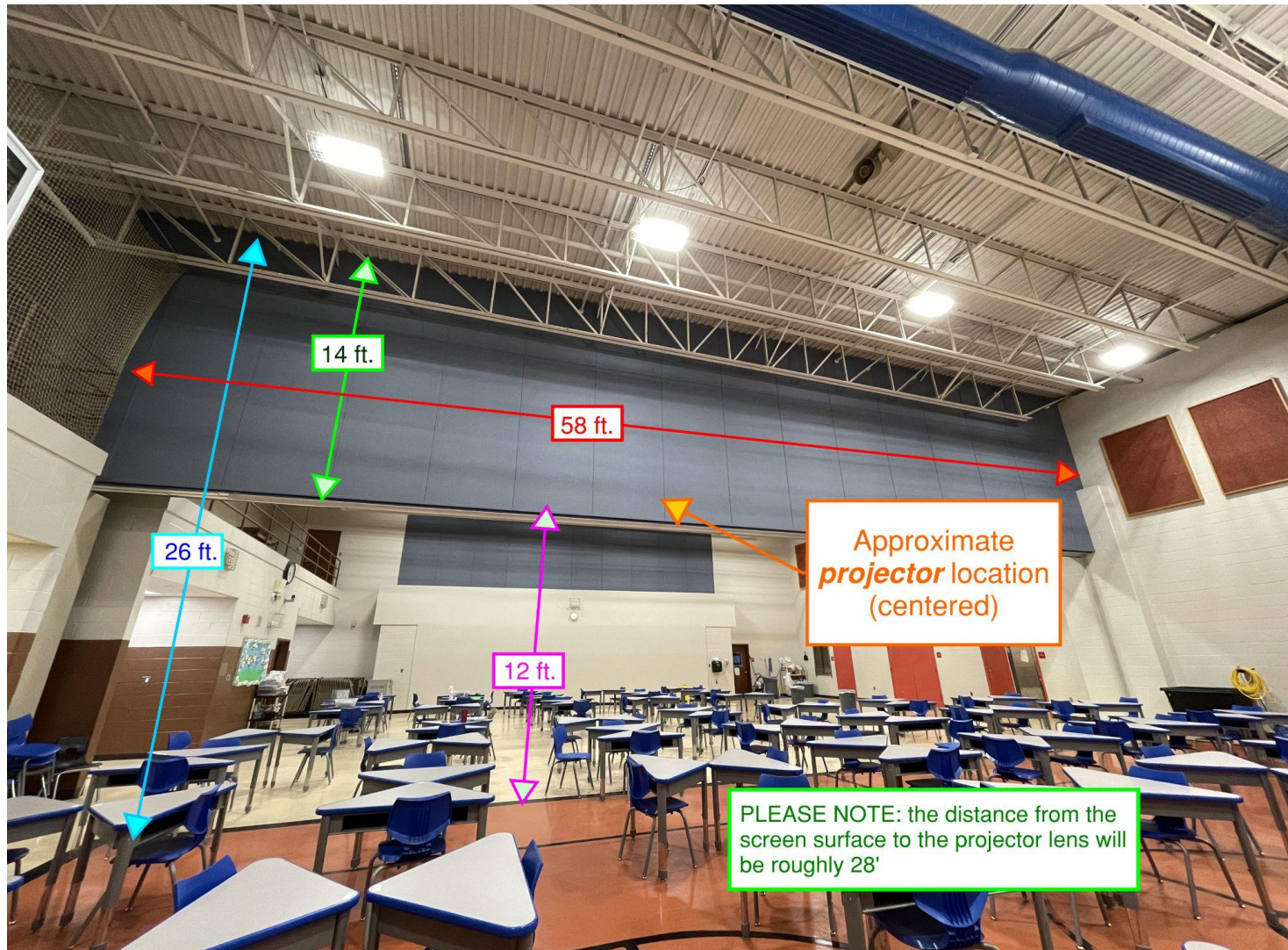
Image #3 - NES Cafeteria Projector Location
